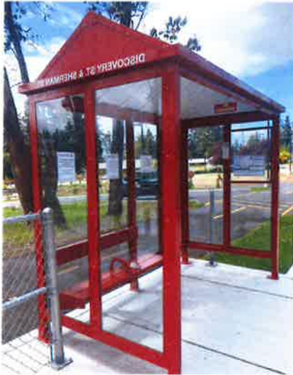
Salish Coast Elementary Bus Shelter
